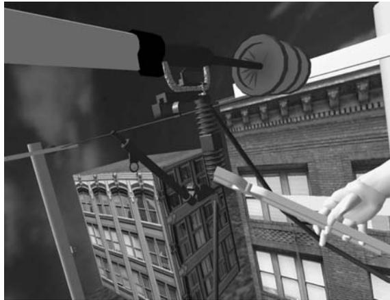
**FIGURE 18** Removal of insulation covers and the end of work.
