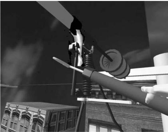
**FIGURE 15** Scene of the fuse holder being closed with the occurrence of an electric spark.
