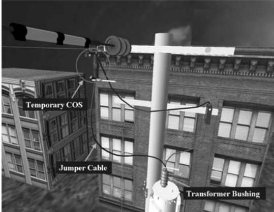
**FIGURE 14** An installed jumper cable between the temporary COS and transformer's first bushing.
