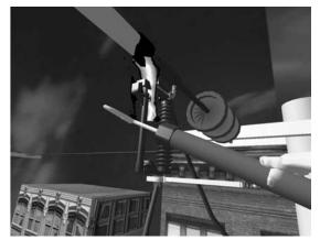
**FIGURE 15** Scene of the fuse holder being closed with the occurrence of an electric spark.
